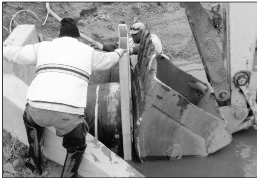
Pallet Push method for installing CheckMate® Valve
