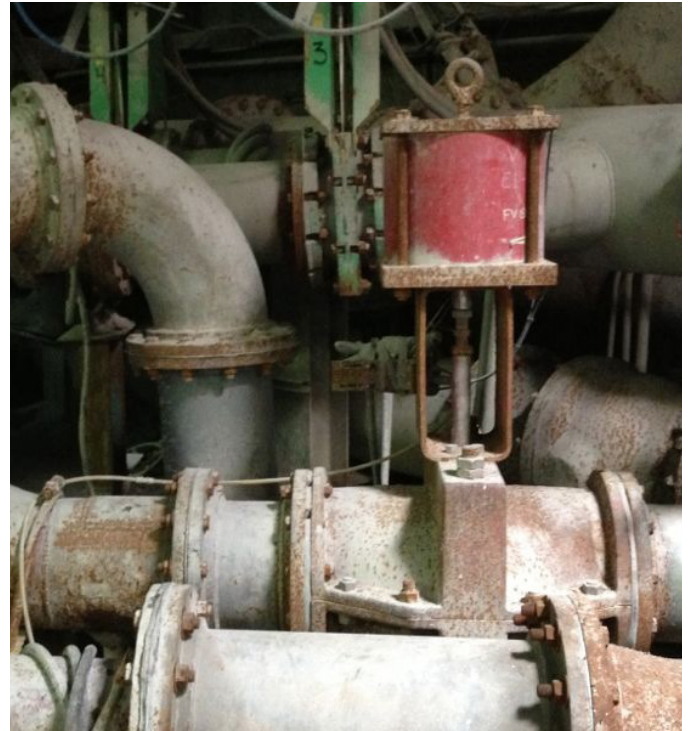
PCV - Series 5200 Control Pinch Valve on a flotation cell tank at a mine in Chile.
